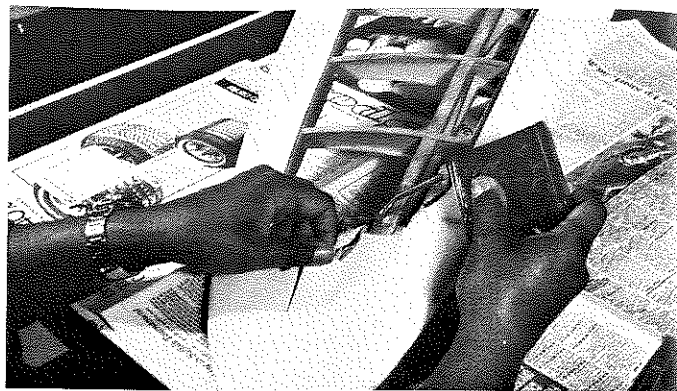
Using thinner to remove planking from top of wing. Note truss bracing between ribs, a typical method of the time.
