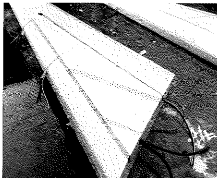
Before the wing cores are sheathed, grooves are cut in the foam with a rotary tool. The wiring harnesses are installed and tested. Afterward, the grooves are filled with foam strips or wood where they add strength.
