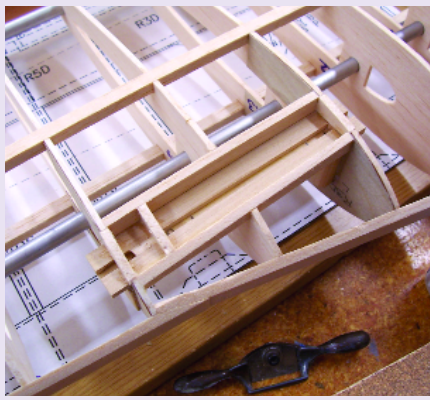
Fully frame and box in the landing-gear blocks before installing the LE sheeting.
