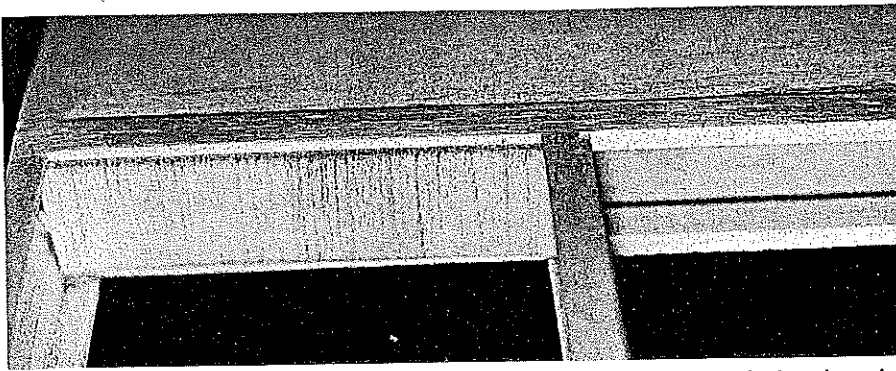
Detail of typical wing spar web (short wing shown here). Note that vertical-grain webs glue against rear face of spars, but are not flush with top or bottom surfaces.
